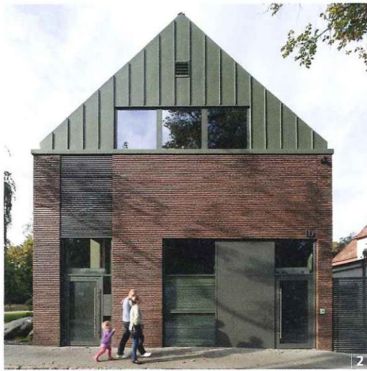
2 | Front elevation. The minimalist body is finished with rusty grey brick and dark grey titanium zinc sheeting. On the left, there is an entrance to the studio, on the right a door leading to flats for rent
